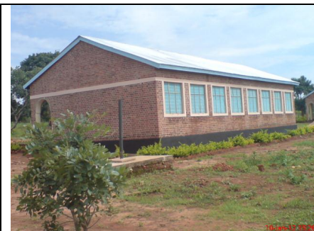
The temporary dormitory building
