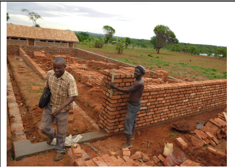
Ntimba and builder working on the new classroom
